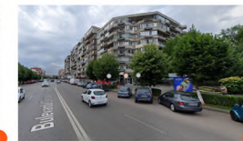
From Bulevardul Decebal view of the Buildings and the road
