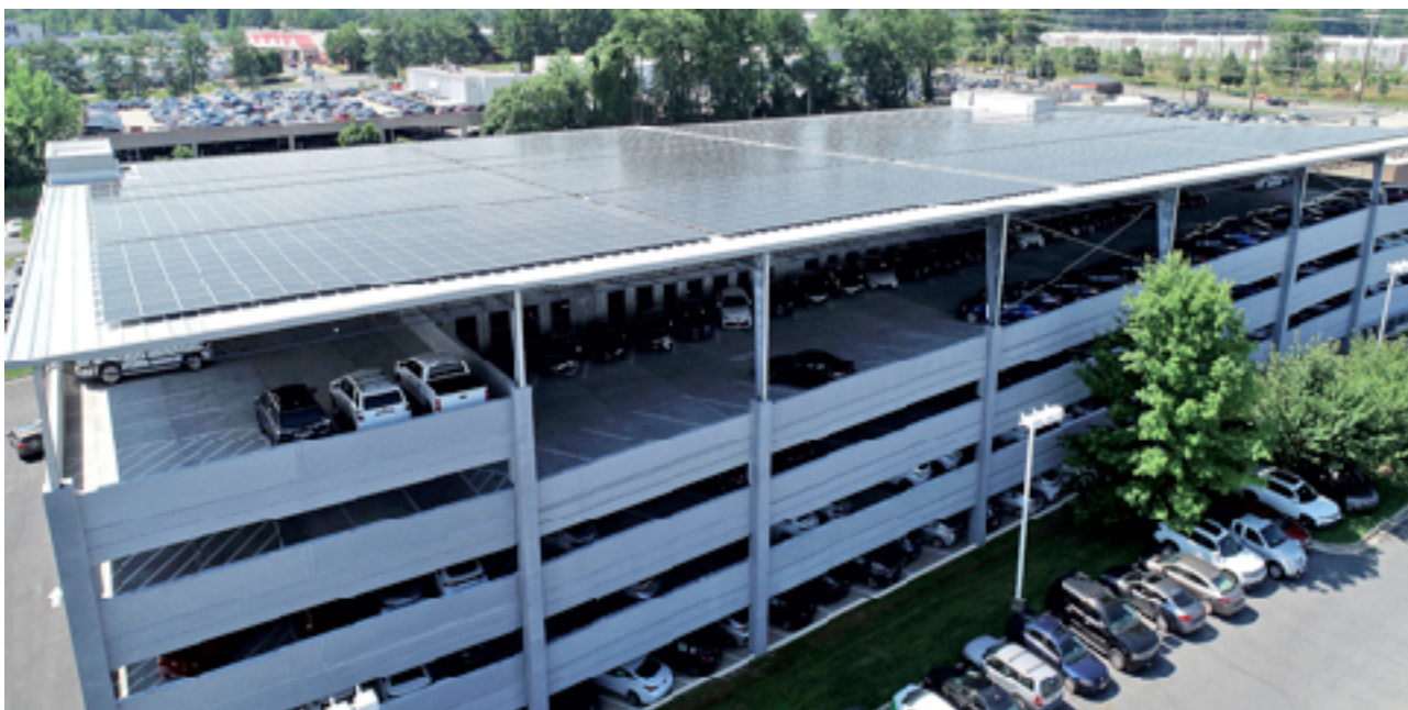
Exemple de acoperire cu panouri fotovoltaice a parcărilor supraetajate. Sursa: https://www.kirbybuildingsystems.com/project-gallery/fitzgerald-parking-garage-solar-canopy-building/
