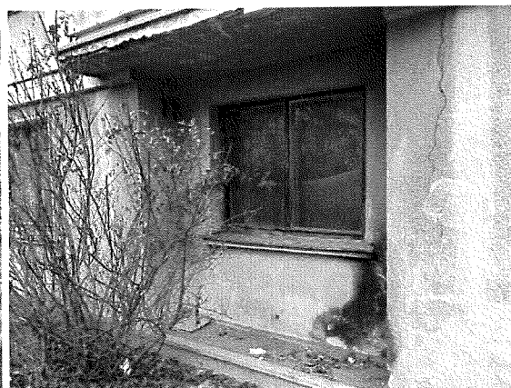
Muchie balcon degradata
